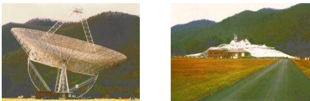
Figure 2. Former 300 foot radio GBT before and after the collapse
