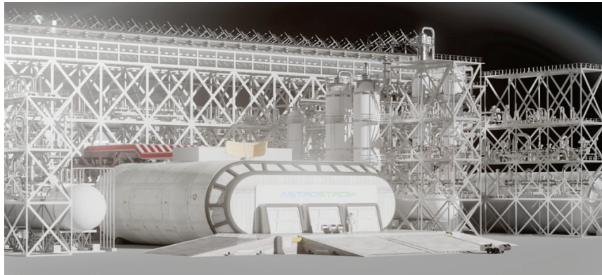
Figure 6: Proposed GE \oplus -LPS beneficiation plant. The basalt racks system allows for modular scalability. (Credit: Astrostrom)
