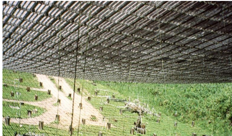
Figure 2-28 Concept of a flat single mesh for GPS layout (credits: INAF)
