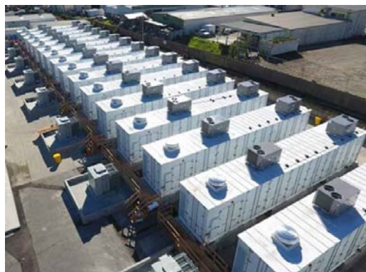
Figure 4-58 EES system installation
