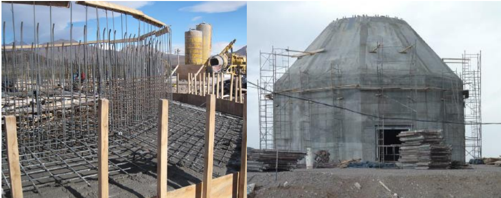
Figure 4.3: Reinforced concrete tower manufactured
