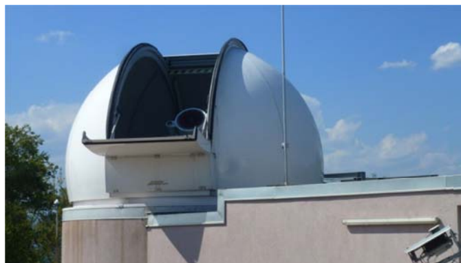
Figure 4-3: The the 5 m diameter dome of the SLR Graz station including a 0.5 m telescope
